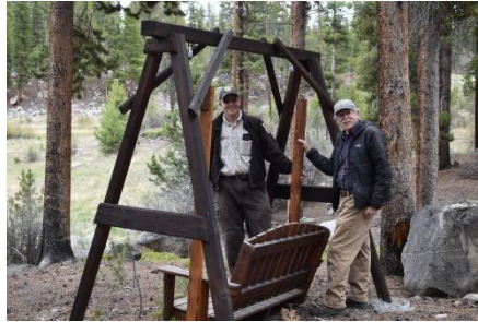
Installing the swing in its new location on Lake 3.
